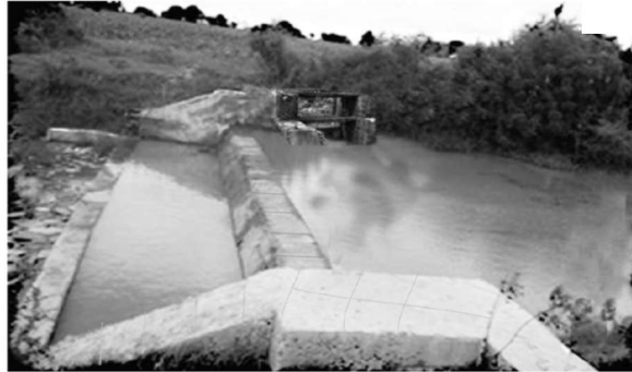
Fig.3 Check Dam with sluice and walkway
